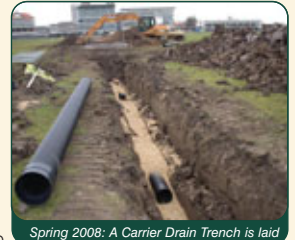
Spring 2008: A Carrier Drain Trench is laid
